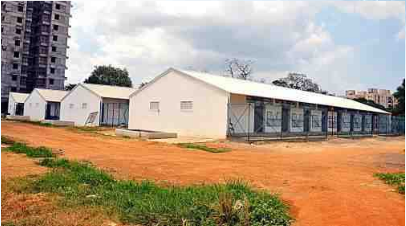
The Newly constructed Stables in the Race Farm.
