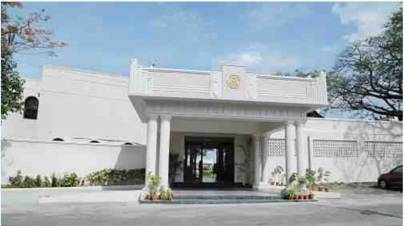
The Newly constructed Entrance to the Paddock / Member Enclosure.
