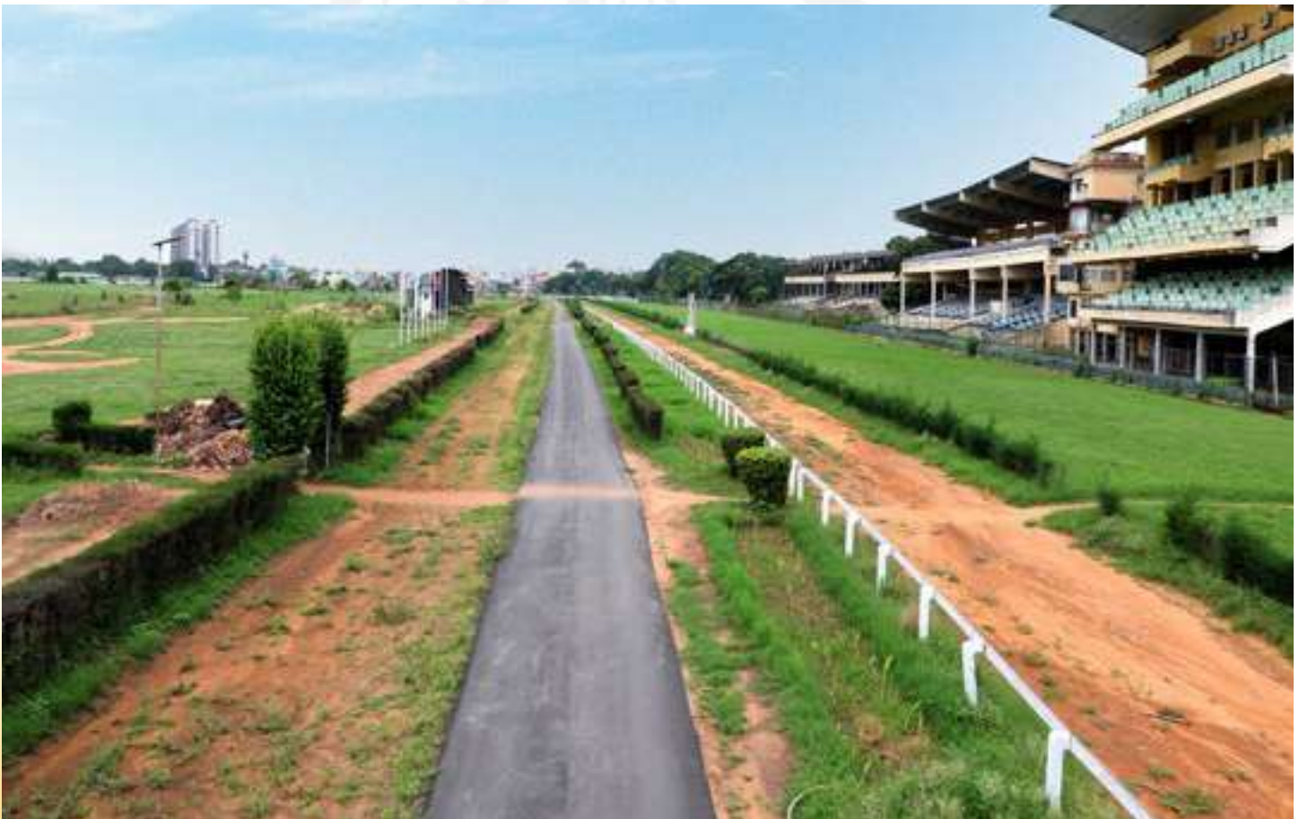
The realigned and asphalted Road inside the Race Course.
